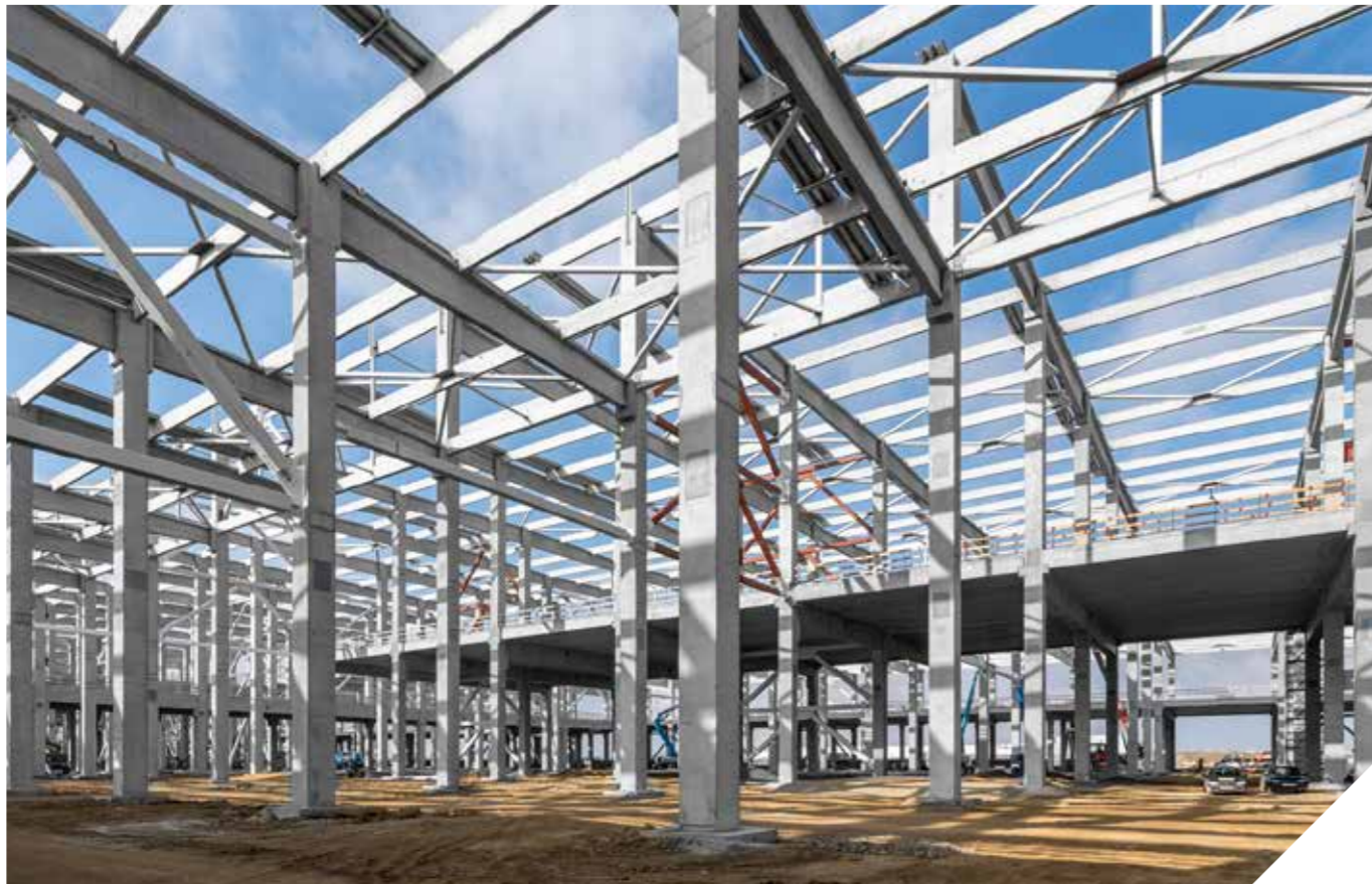
CATL, Debrecen Year of handover: 2022.. Delivered products: complete prefabricated structure Floor area: 23.890 m 2 Produced quantity: 3.945 m 3
