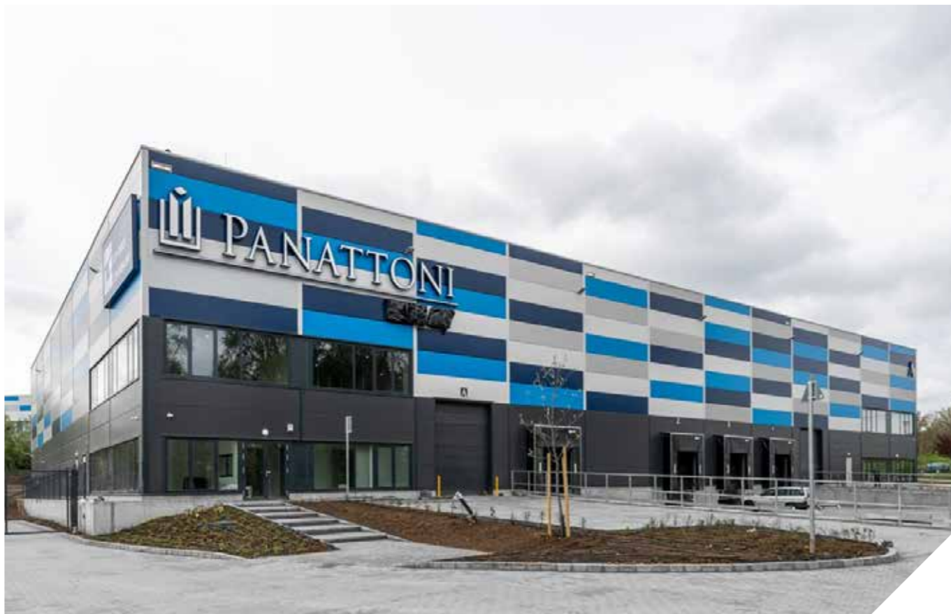
Panattoni City, Törökbálint Year of handover: 2023. Delivered products: complete prefabricated structure Produced quantity: 2.130 m 3
