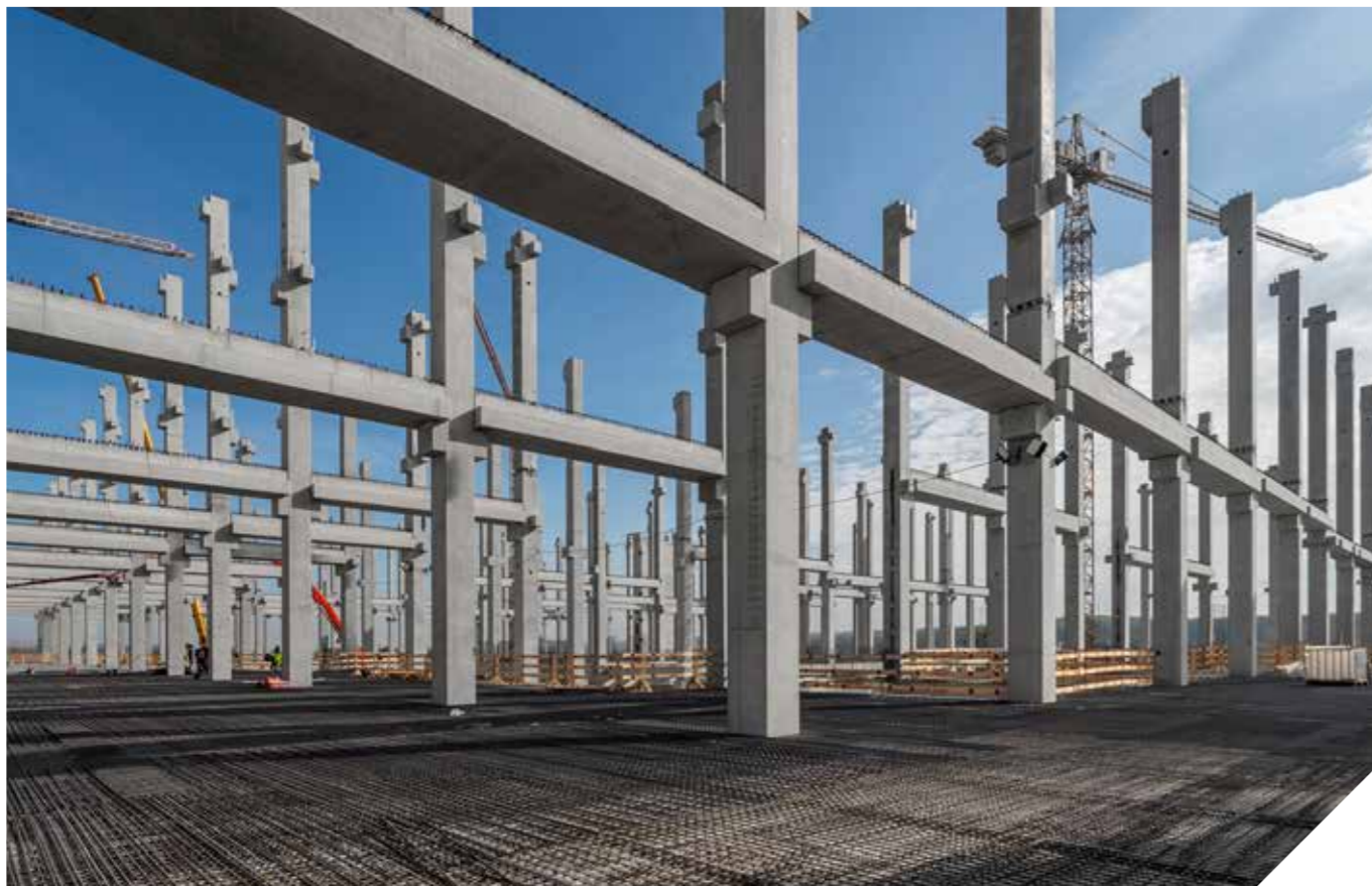
BAMO-Cobalt, Ács Year of handover: 2025. Delivered products: complete prefabricated structure Floor area: 15.876 m 2 Produced quantity: 3.730 m 3
