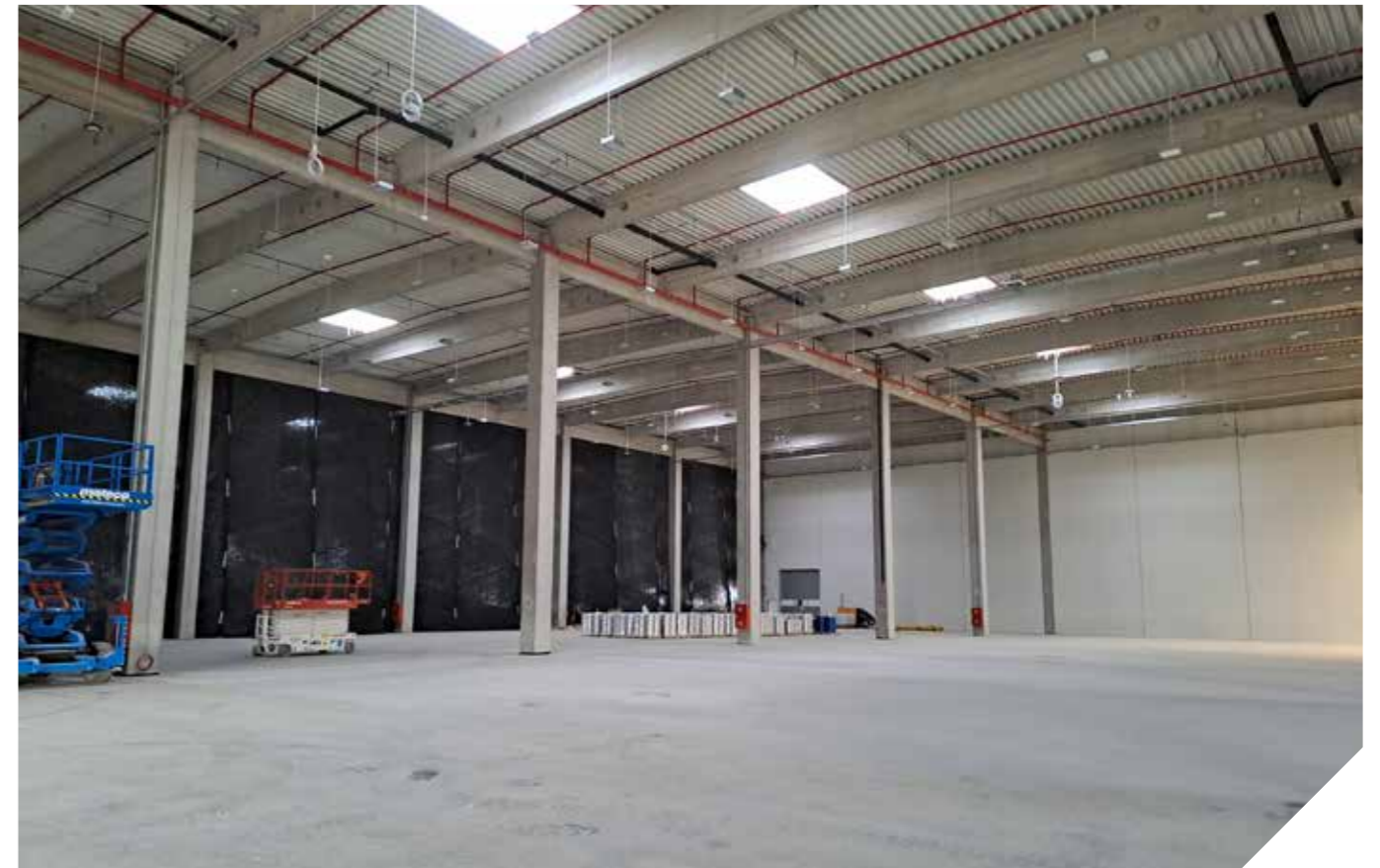
Inpark, Debrecen Year of handover: 2023.. Delivered products: complete prefabricated structure Floor area: 73.000 m 2 Produced quantity: 11.377 m 3
