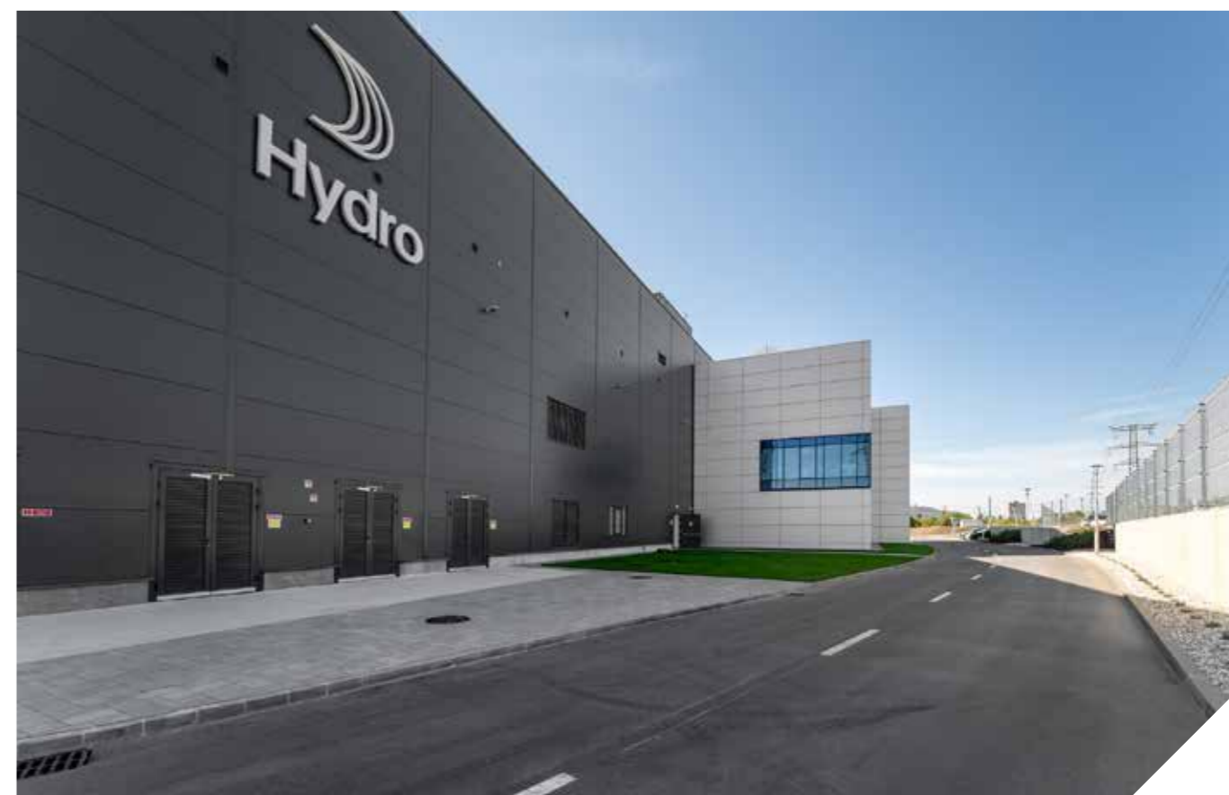
HYDRO Aluminum foundry and office, Székesfehérvár Year of handover: 2023. Delivered products: complete prefabricated structure Floor area: 21.000 m 2 Produced quantity: 3.540 m 3
