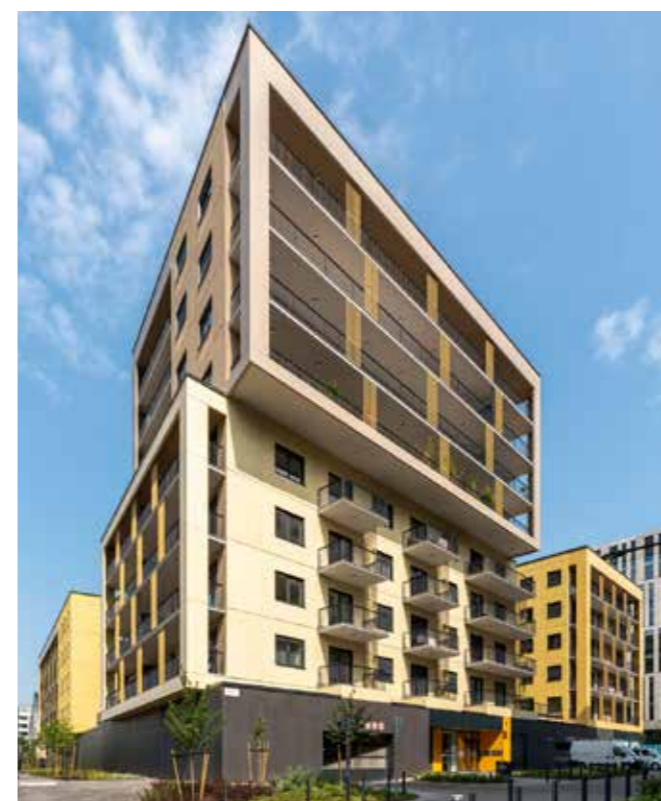
BudaPart - BOG Hotel and Office, BRF, BRG, BOA, BOIJ, BOH, BOK, BOL, BOM, BRK, BRL Year of handover: 2022 – 2025. Delivered products: prefabricated sandwich wall panels, stairs, balcony, cover sheets, retaining walls
