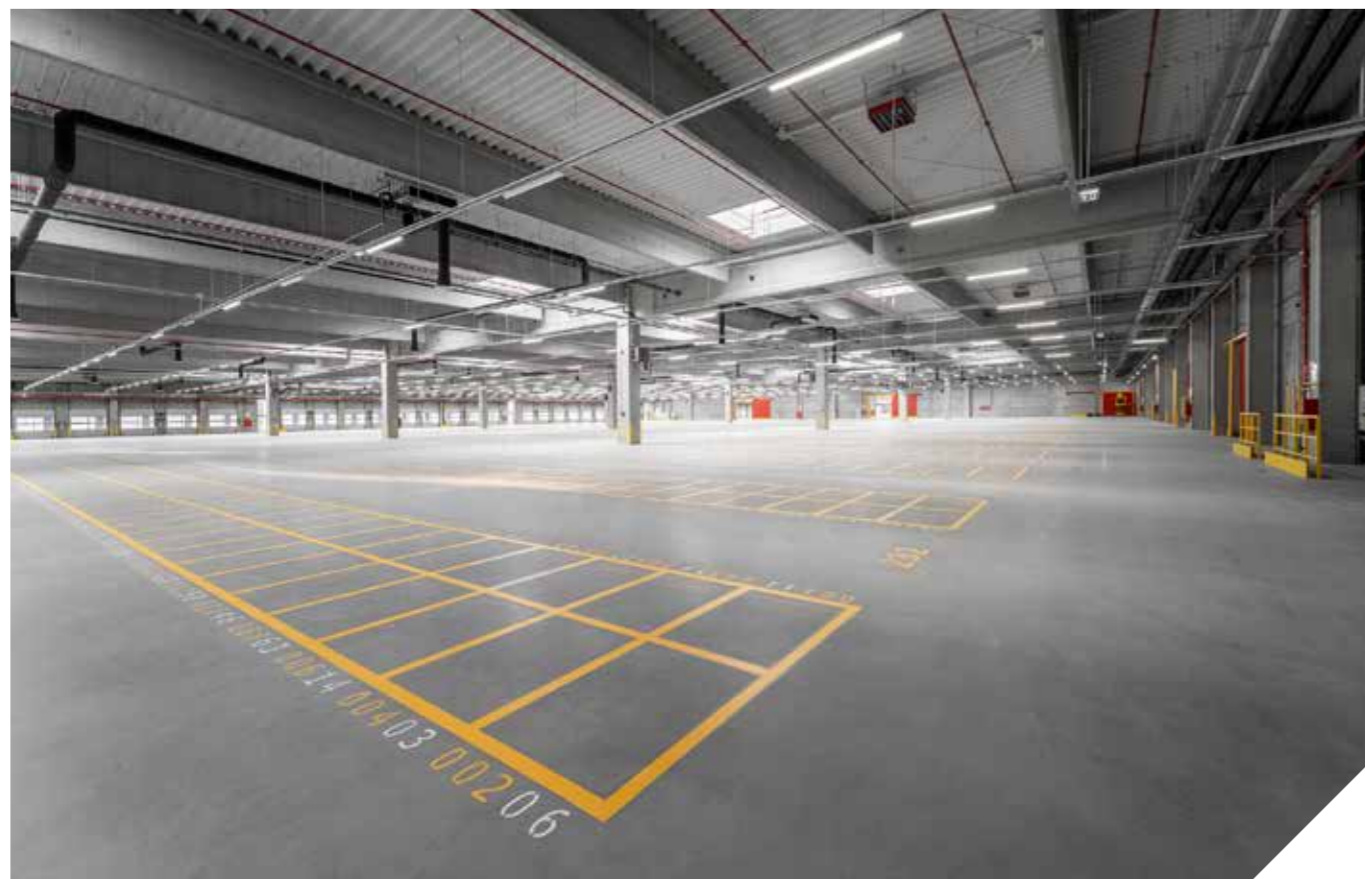
JYSK DCE Logistics Center, Ecsér Year of handover: 2021. Delivered products: complete prefabricated structure
