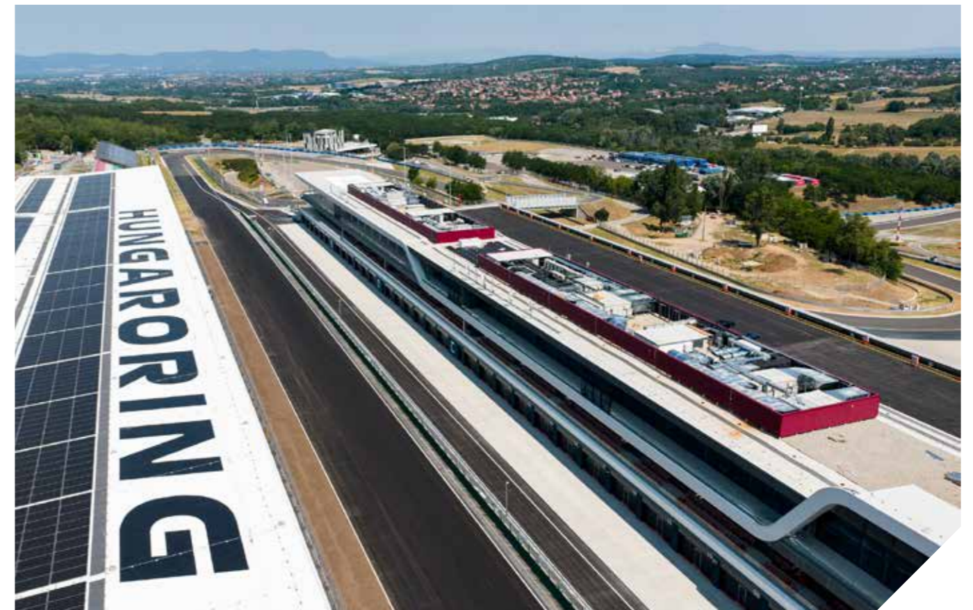
HUNGARORING – Depó, Paddock, Grandstand, Event space, Mogyoród Year of handover: 2025. Delivered products: complete prefabricated structure Produced quantity: 2.492 m 3 Grandstand elements: 1.671 m 3
