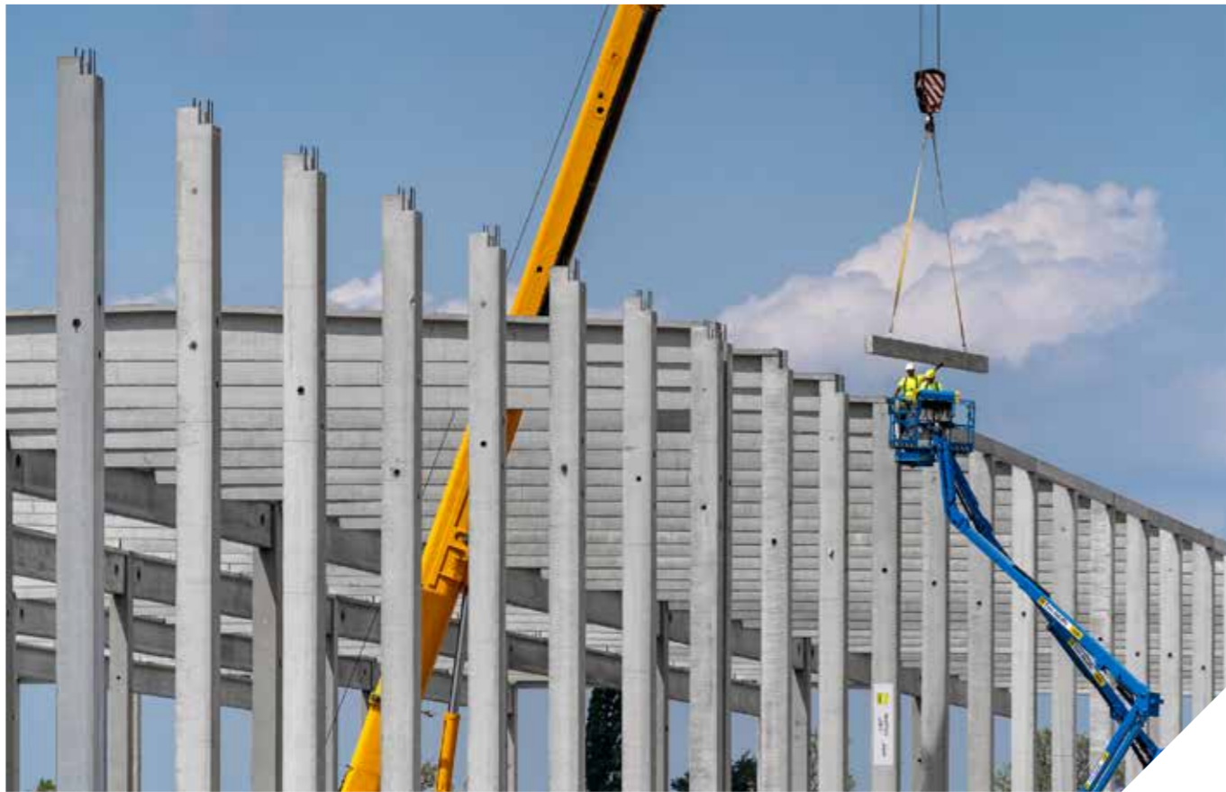
HelloParks MG3, Maglód Year of handover: 2023. Delivered products: complete prefabricated structure Floor area: 46.000 m 2 Produced quantity: 3.630 m 3
