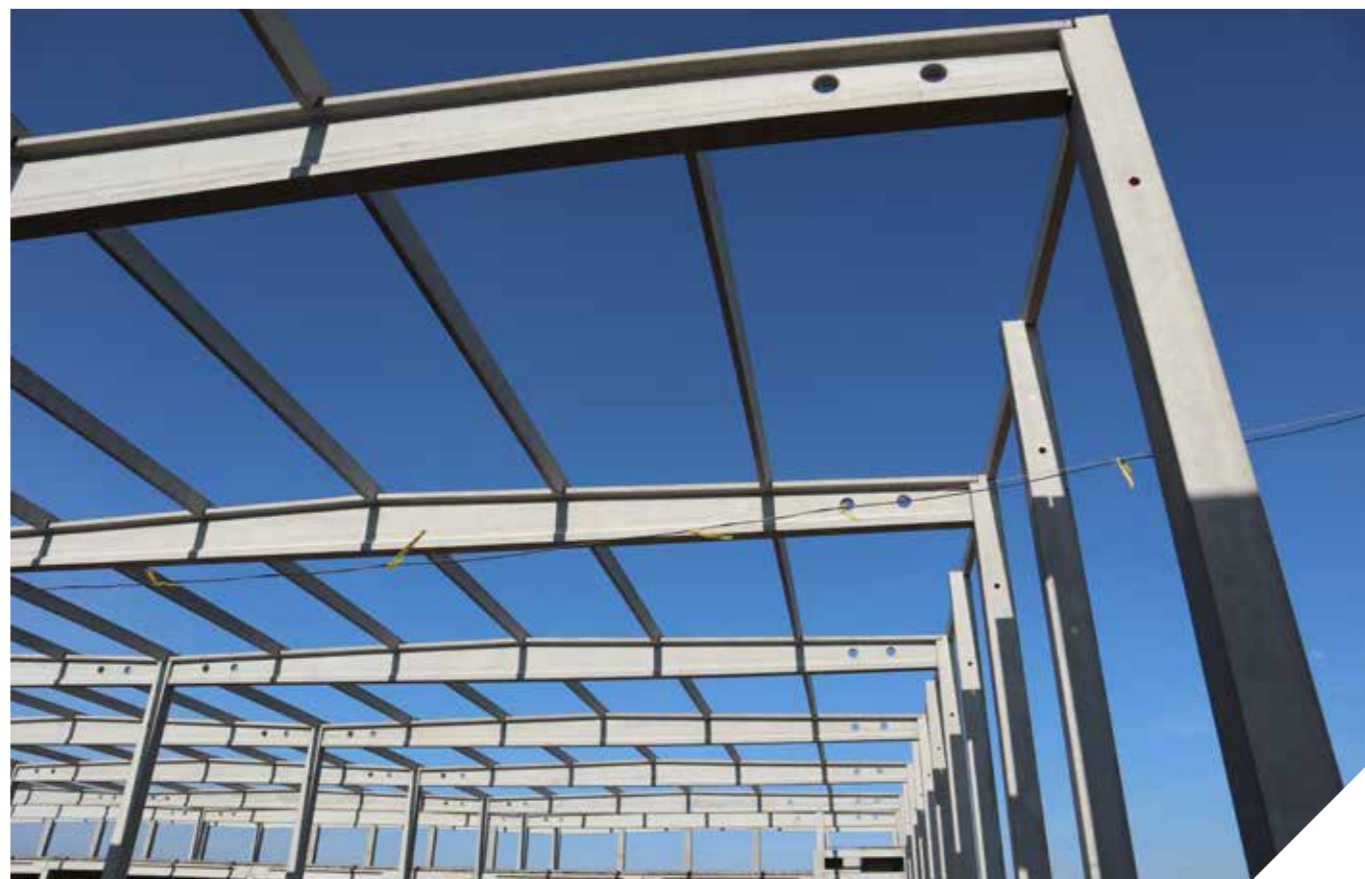
Horváth Rudolf Intertranszport Kft., Hatvan Year of handover: 2024. Delivered products: 2 complete prefabricated structure Floor area: 40.000 m 2 Produced quantity: 4.375 m 3
