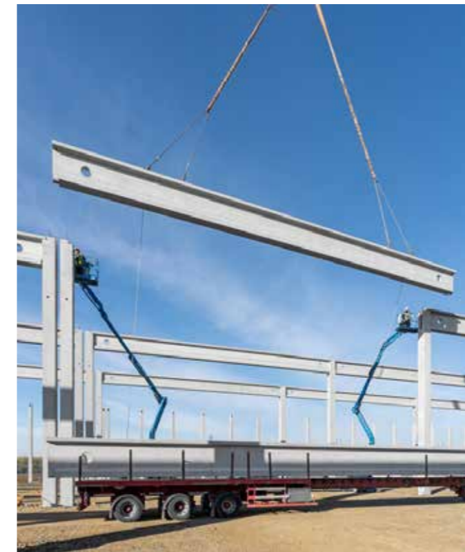
HelloParks MG4, Maglód Year of handover: 2023. Delivered products: complete prefabricated structure Floor area: 45.500 m 2 Produced quantity: 4.270 m 3
