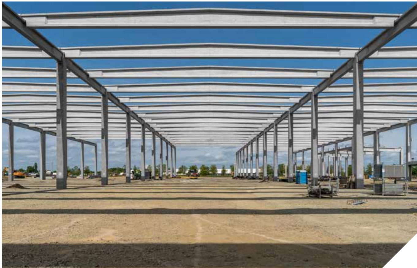
Benepack, Makó Year of handover: 2024. Delivered products: complete prefabricated structure Produced quantity: 3.642 m 3
