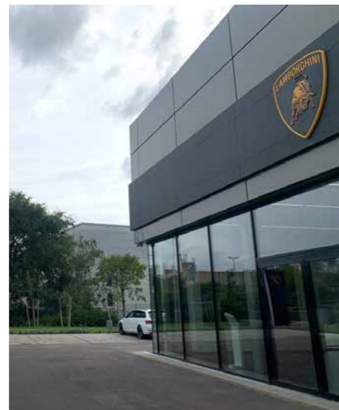
Lamborghini Car Showroom, Budapest Year of handover: 2023. Delivered products: complete prefabricated structure Floor area: 635 m 2 Produced quantity: 73 m 3
