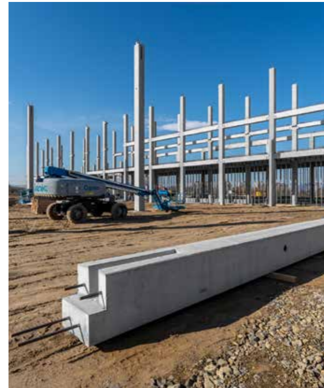
Euromedic, Budapest Year of handover: 2024. Delivered products: complete prefabricated structure Floor area: 11.800 m 2 Produced quantity: 1.564 m 3
